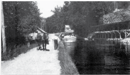
The barge has just left Lock No. 9, north of New Paltz, New York, on the Delaware and Hudson Canal.
