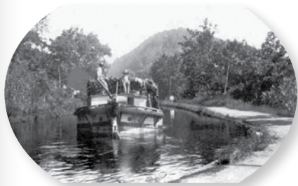
After leaving Lock No. 8, the barge loaded with firewood continues northeast towards Rosendale, New York. The man on the left is steering the barge. The mules towing the barge are in the distance on the towpath. The above photos taken by William or John Crabtree in the late 1800s are courtesy of The Century House Historical Society.
